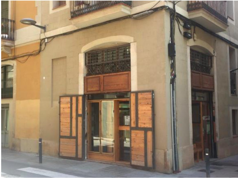
Photo 1: Front of building Lacol
