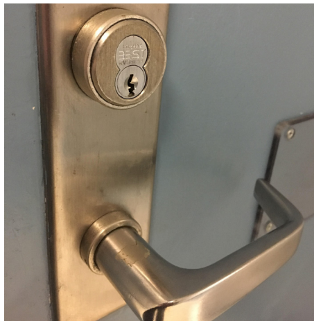
PRINTED WITH PERMISSION FROM M. RINKA NSU plans to improve safety by changing all the locks in the residence halls.
