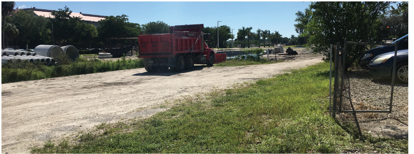
Construction of the new Southwest 36th Street.
