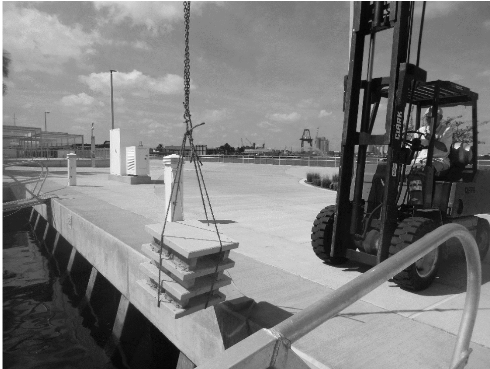
Figure 3. Artificial reef modules were deployed into the NSU-GHOC boat basin by forklift. A diver in the water assisted with module placement.
