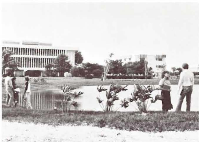
Looking across Gold Circle Pond toward the Mailman-Hollywood Building and the Family Center.
