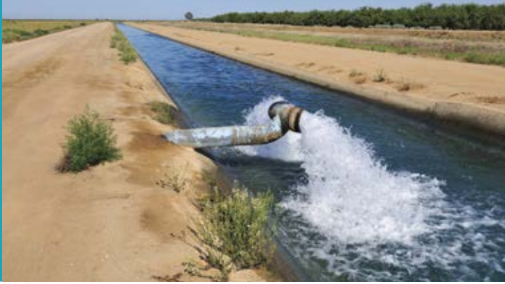
Irrigation canal and valve, California, USA. Source: Richard Thornton
