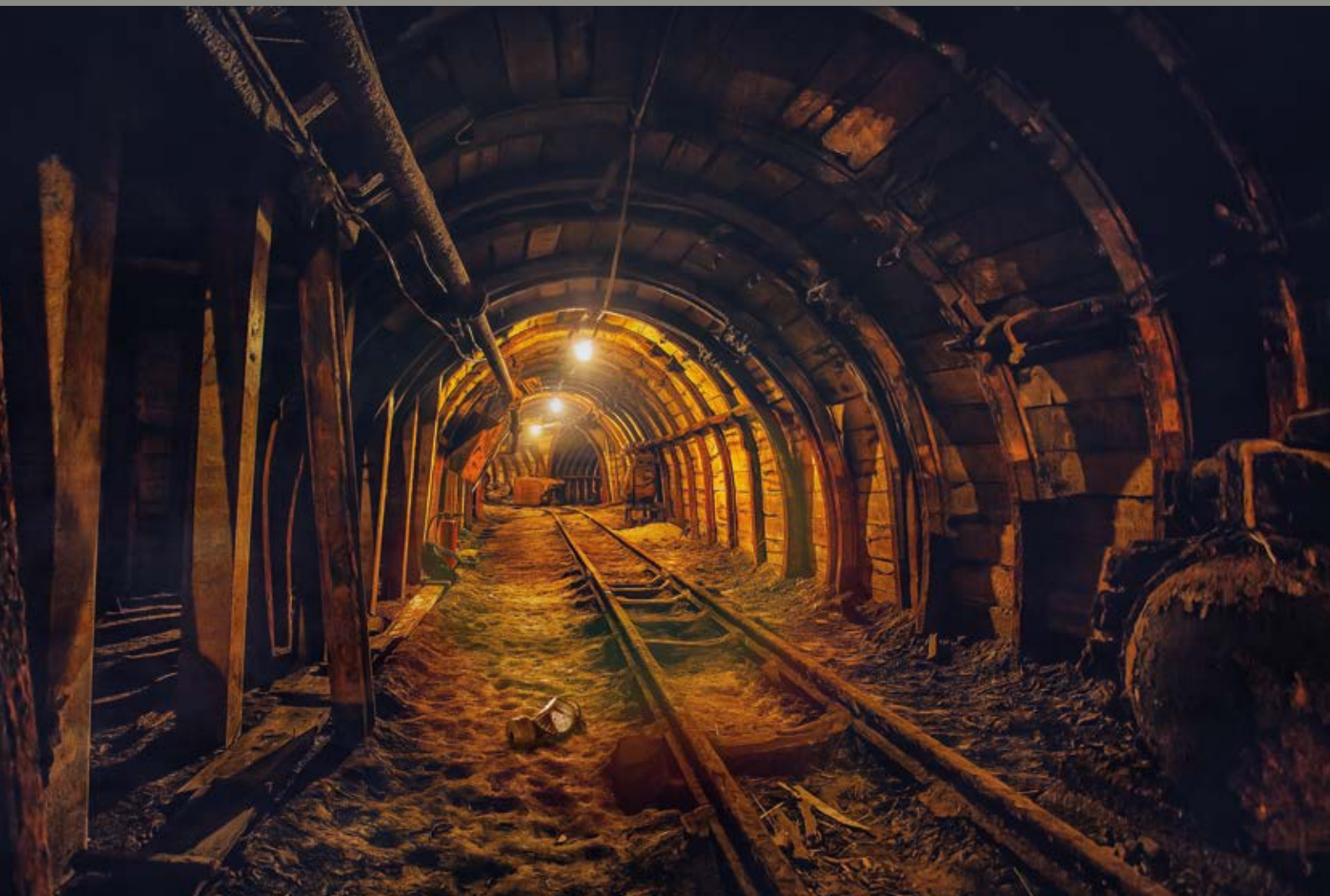
Underground mine tunnel.
