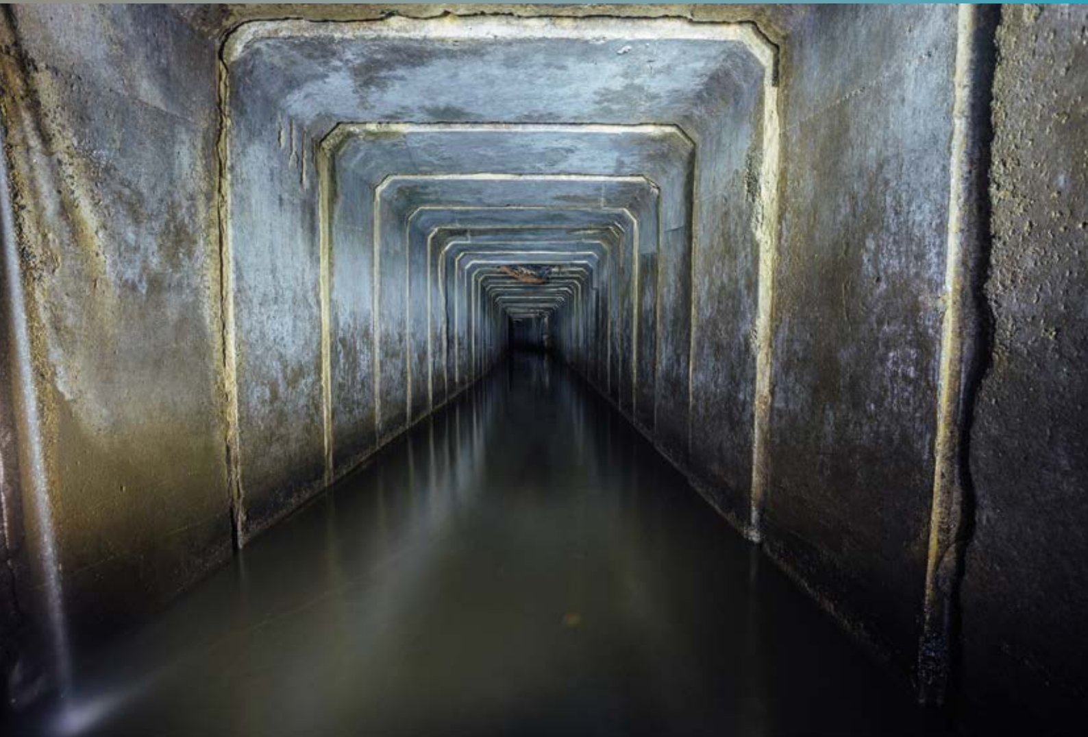
'Blue Danube' subterranean sewer tunnel, Voronezh, Russia.
