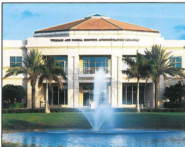
Nova Southeastern University's Administration Building, Fort Lauderdale, Florida
