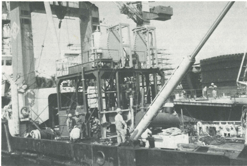
Closeup view of the ship used by the Japanese OTEC team in recent experiments. Note the heat exchangers, top center.
