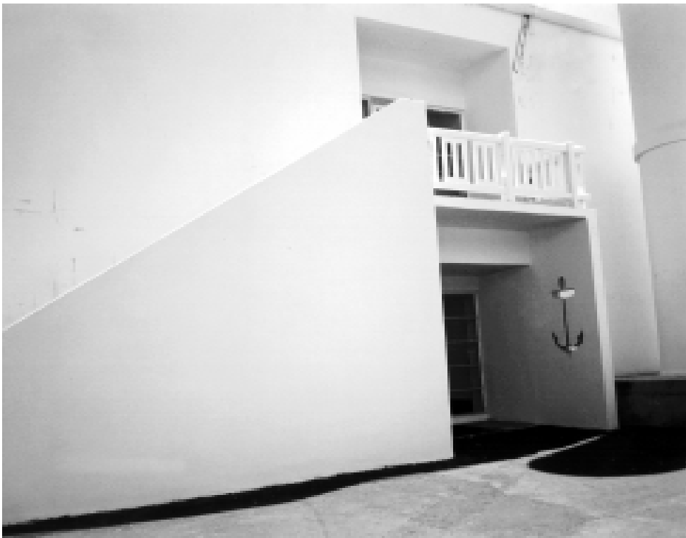
Sleek new stairway and entrance to Forman Building
