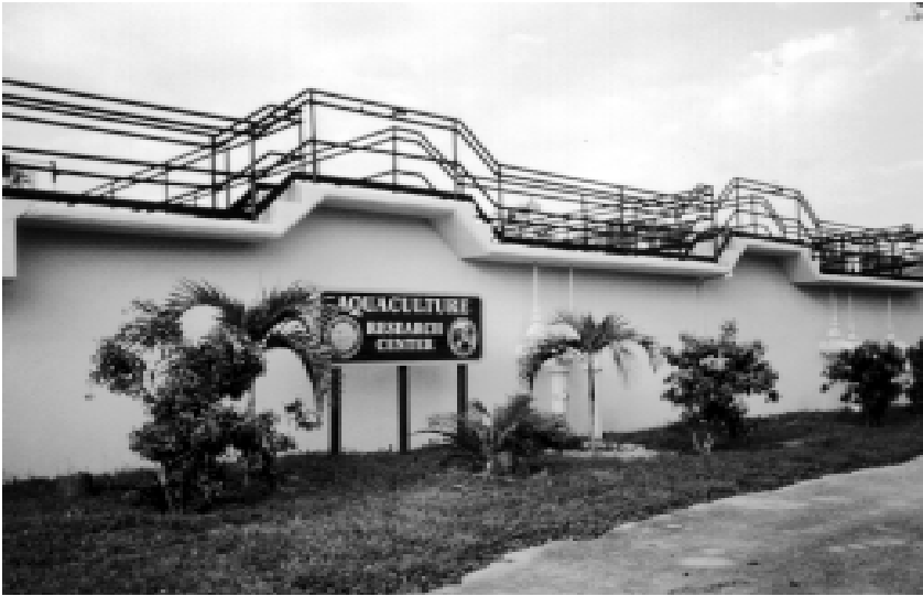
Davie aquaculture facility
