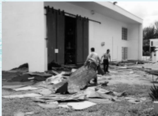
Fixing the roof after Irene
