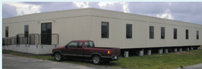
The new modular was set up on the site of the old trailer.
