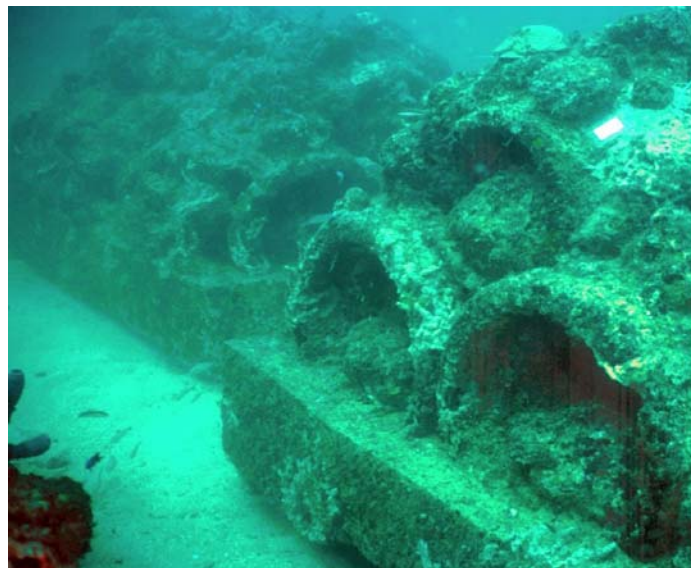
Figure 5: DERM Module utilized as artificial reef (Monty, 2006).
